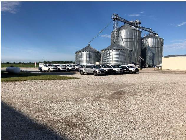
Grain storage facilities at the site of the Fumigation Workshop
