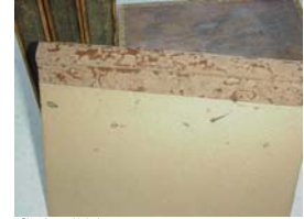
Example of Silverfish Damage
