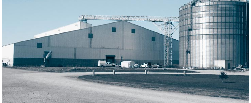
11.5 million cubic foot corn flat storage fumigated with phosphine.
